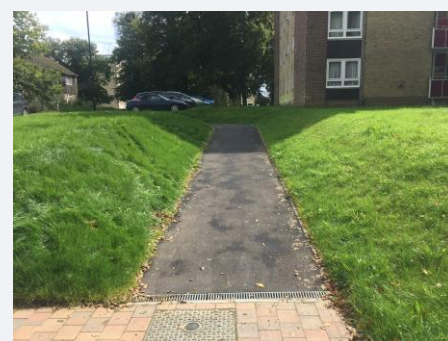
New Access Ramp to Flats
